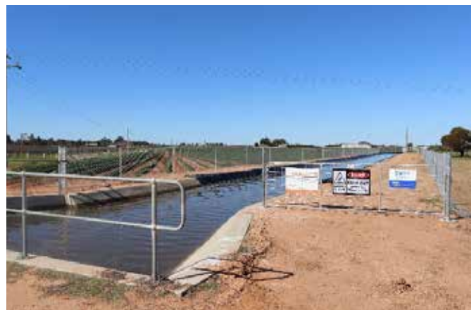
Above: Channel lining works completed this winter at Red Cliffs
