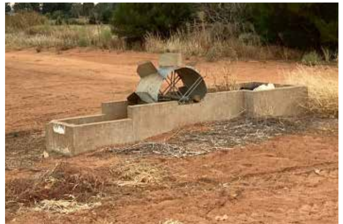
Above: A Dethridge wheel to be removed as part of the SWEP.
