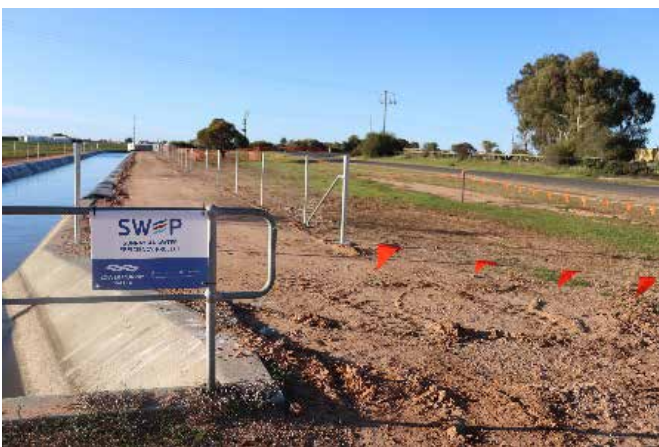
Above: Channels lined under SWEP have been fenced to improve safety.
