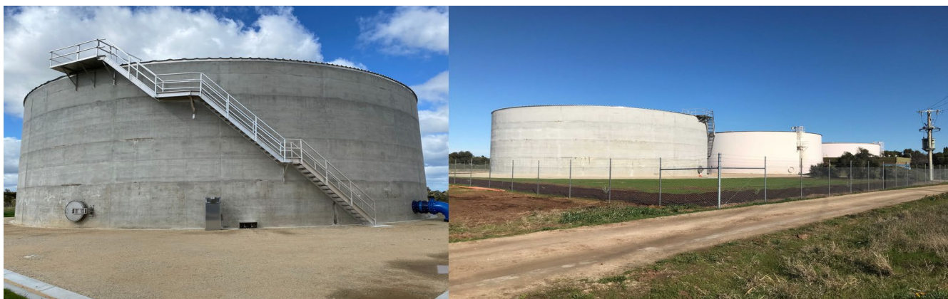
Figure 2 New 5 ML storage tank in Swan Hill
