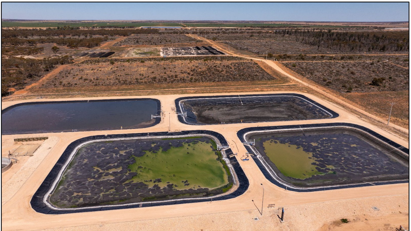
Image 4: Koorlong Waste Water Treatment Plant
