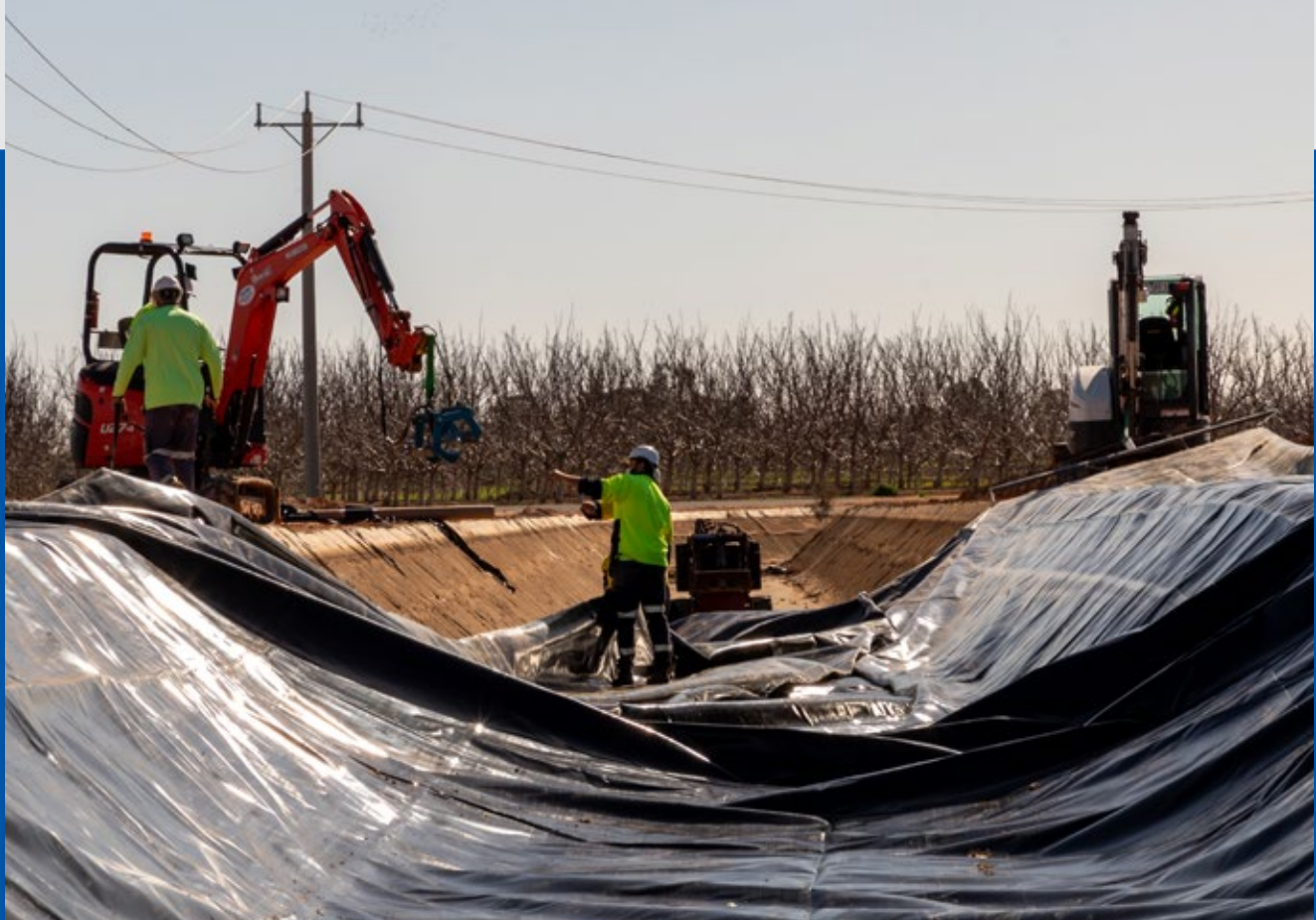
Channel Lining - Winter Maintenance Works, Red Cliffs
