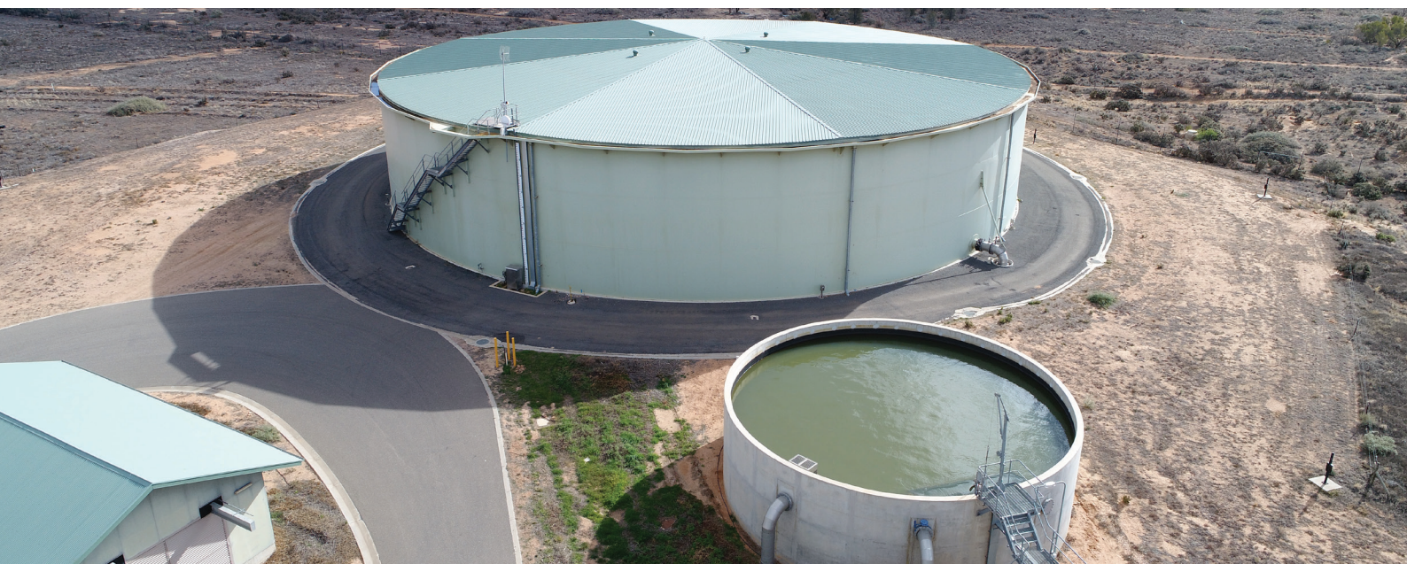
Mildura West Water Treatment Plant.
