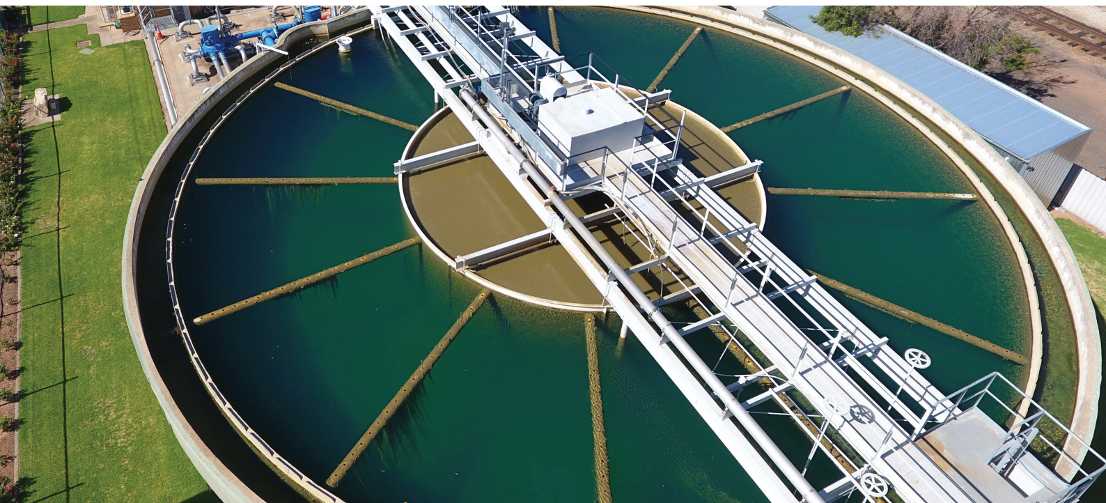
Swan Hill Water Treatment Plant
