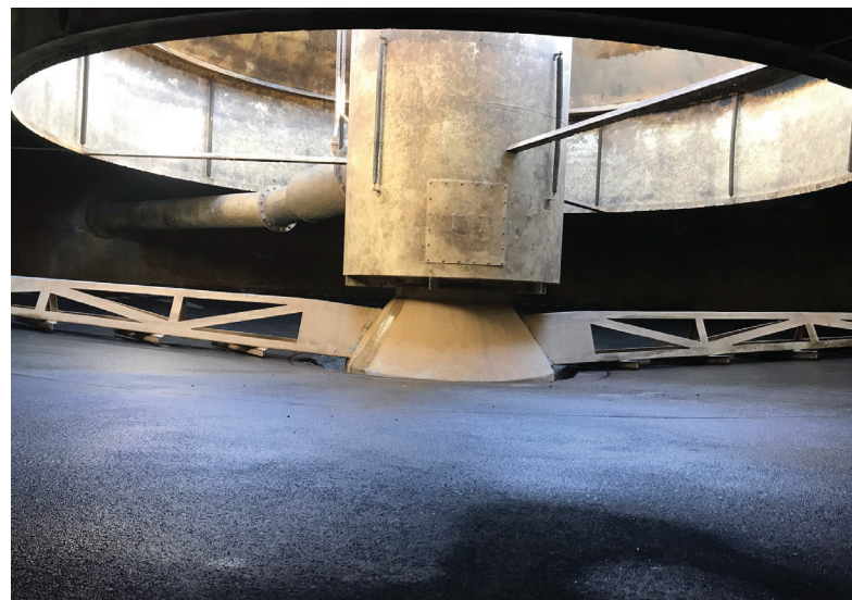
Inspection of clarifier No. 3 at Mildura Water Treatment Plant
