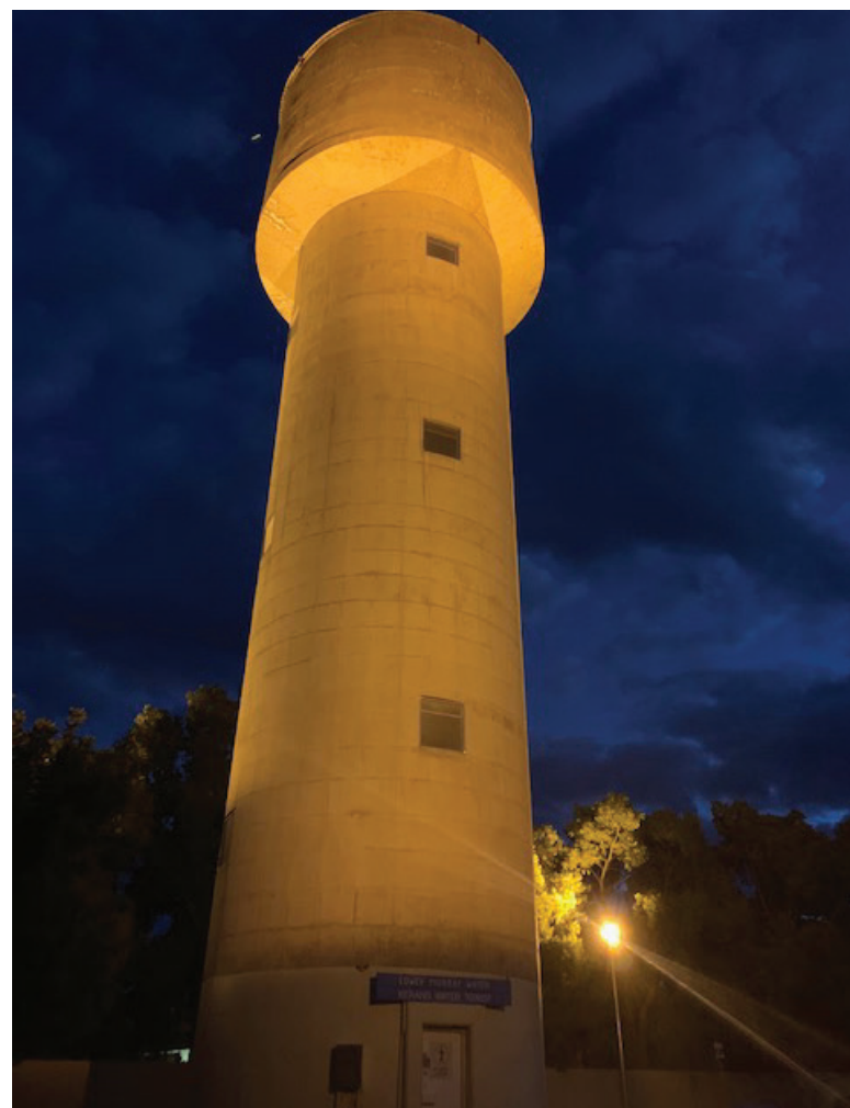
Kerang Water Tower
