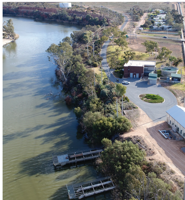
Red Cliffs Water Treatment Plant and Irrigation Pump Station
