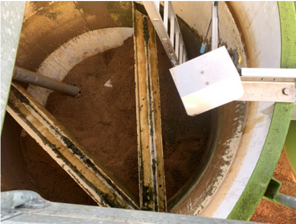
Figure 2 - Removal of filter media from Robinvale WTP Filter #1
